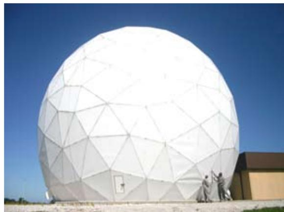
The giant golf ball, as it's known at MacDill, is actually a protective covering for the "giant" communications satellite dish inside it at the STEP facility. The dome protects the dish from the elements, and also conceals the direction the dish is pointed to ensure operations security.
