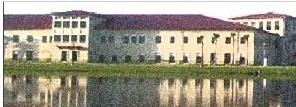
The 6th Medical Group headquarters and clinic is the first major structure encountered by visitors to MacDill Air Force Base.
